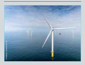
The Dudgeon Offshore Wind Farm is situated between 20 to 32 miles off the coast of Cromer in North Norfolk. It consists of 67 wind turbine generators (6MW) and produces sufficient electricity to power around 410,000 UK homes.
